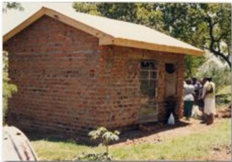
Figure 15. Mushroom house made of earthen bricks, cement walls and iron sheet roof.
