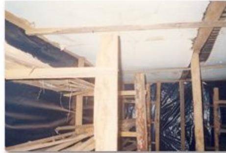
Figure 12. Roof insulated with cartons
